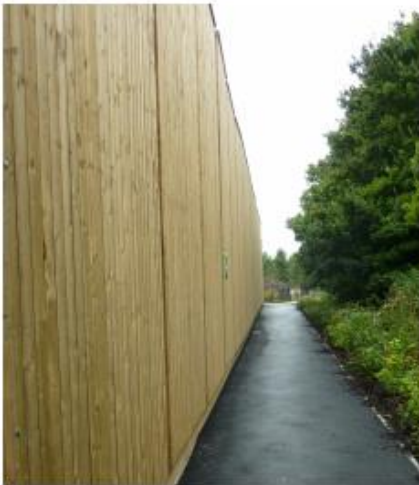
ACOUSTIC FENCE DETAIL
